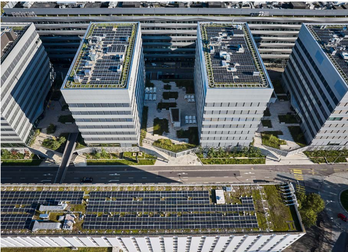
Stücki Park in Basel, completed in 2024, was constructed to the very latest sustainability requirements (here an aerial view of photo-voltaic systems on the roofs).
