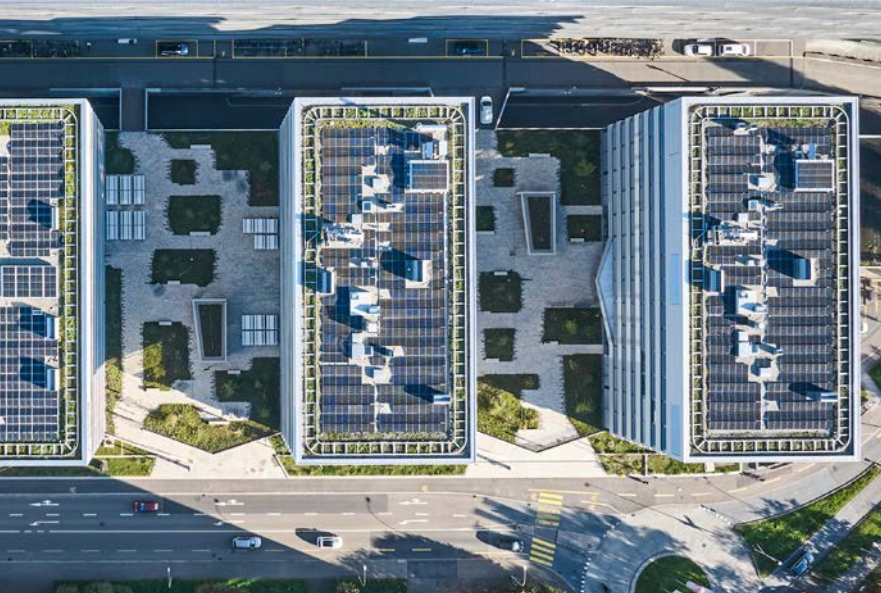
Photovoltaic system, Stücki Park Basel
