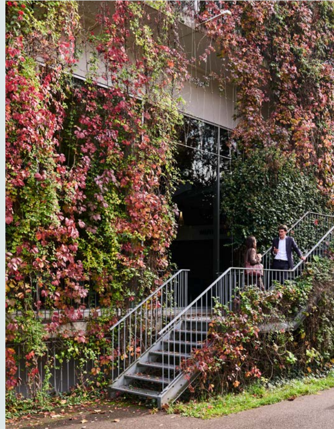
Green façade, Stücki Park in Basel
