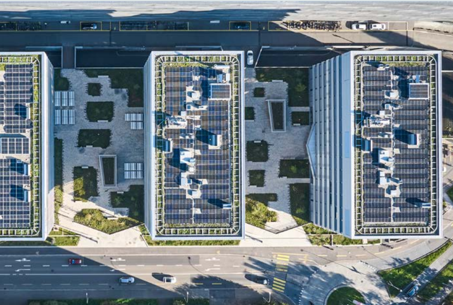
Photovoltaic system, Stücki Park Basel
