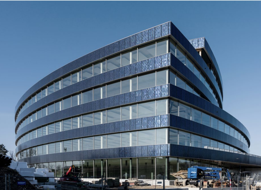
BERN 131, Berne, with façade cladding consisting of photovoltaic modules
